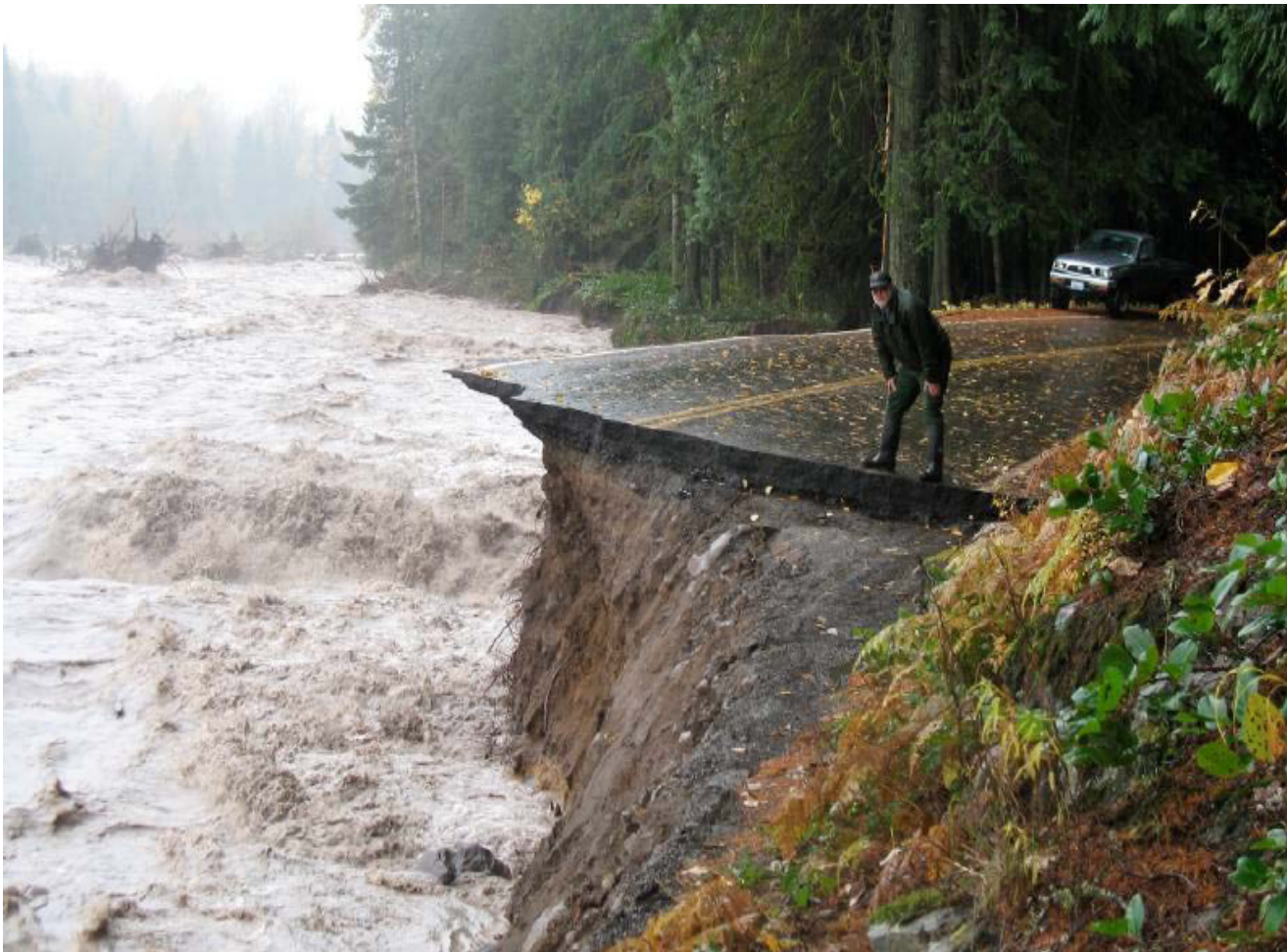
Nisqually River at Sunshine Point (Nov, 2006)
